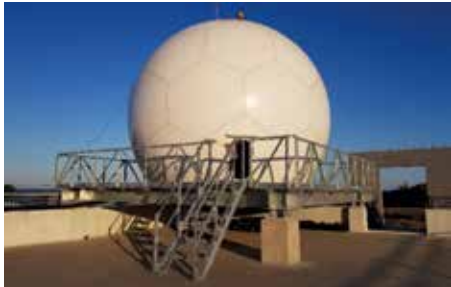
Jeju ground station
