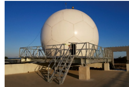
Jeju ground station
